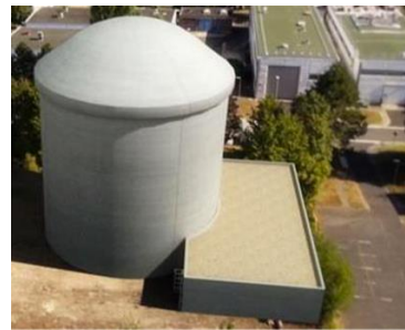
VERCORS mock-up: containment building at scale 1:3
